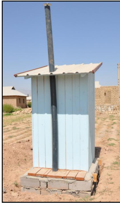
Photo 1: Save the Children Sanitation Block made of timber frame /porous concrete blocks
