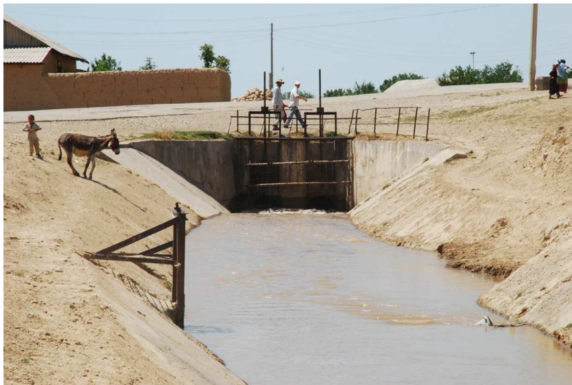
Figure 4: Open irrigation channel above the agricultural fields to the west of Uyali. Clearly visible is the beginning of the underground pipes that run several hundred meters downhill. Picture taken on June 17 th .
