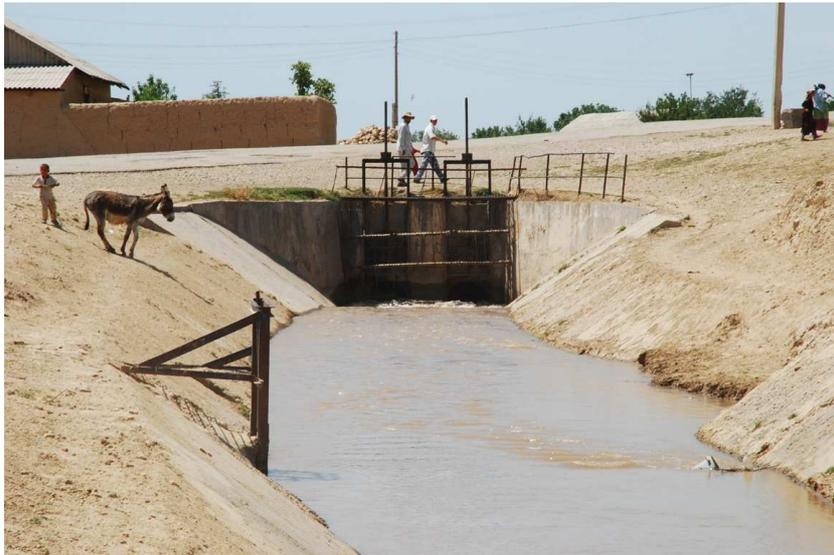
Figure 4: Open irrigation channel above the agricultural fields to the west of Uyali. Clearly visible is the beginning of the underground pipes that run several hundred meters downhill. Picture taken on June 17<sup>th</sup>.
